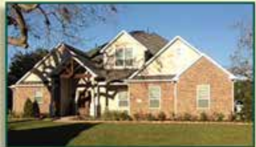
Custom Home just completed on our client's lot in Weston Lakes
